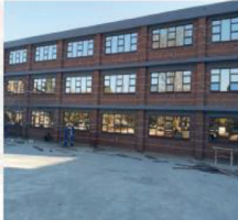
Final touches to the Innovation Hub at the University of Zimbabwe
