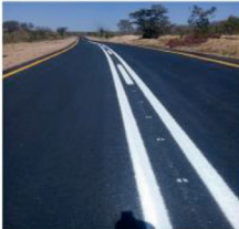
Completed section of the Bindura-Matepatepa Road
