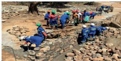
Mhakwe Causeway reconstruction in progress. (Chimanimani District)
