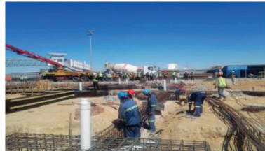
Expansion of Harare International Airport
