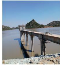
Upstream View of Marovanyati Dam
