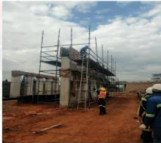
Ongoing works on the Norton Road Over Rail Bridge
