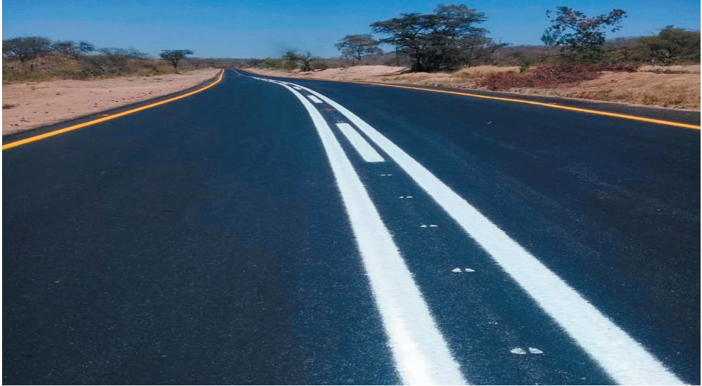
Completed section of the Bindura-Matepatepa Road
