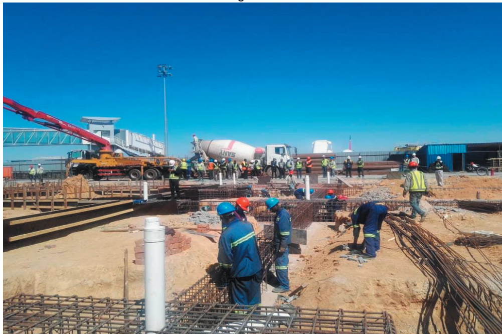
Work on foundations for terminal building extension
